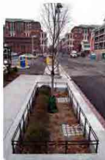
A lowered roadside swale in Washington, D.C. absorbs and naturally filters water collected from the street. Photo courtesy of Chesapeake Bay Program
